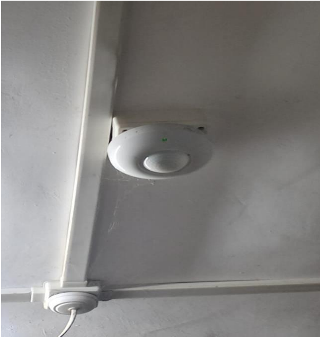
Light sensing circuit
